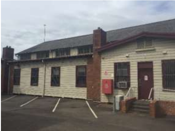
Army training hall in southeast corner of site with plaque indicating structure was built in 1910. Note asbestos roof.
